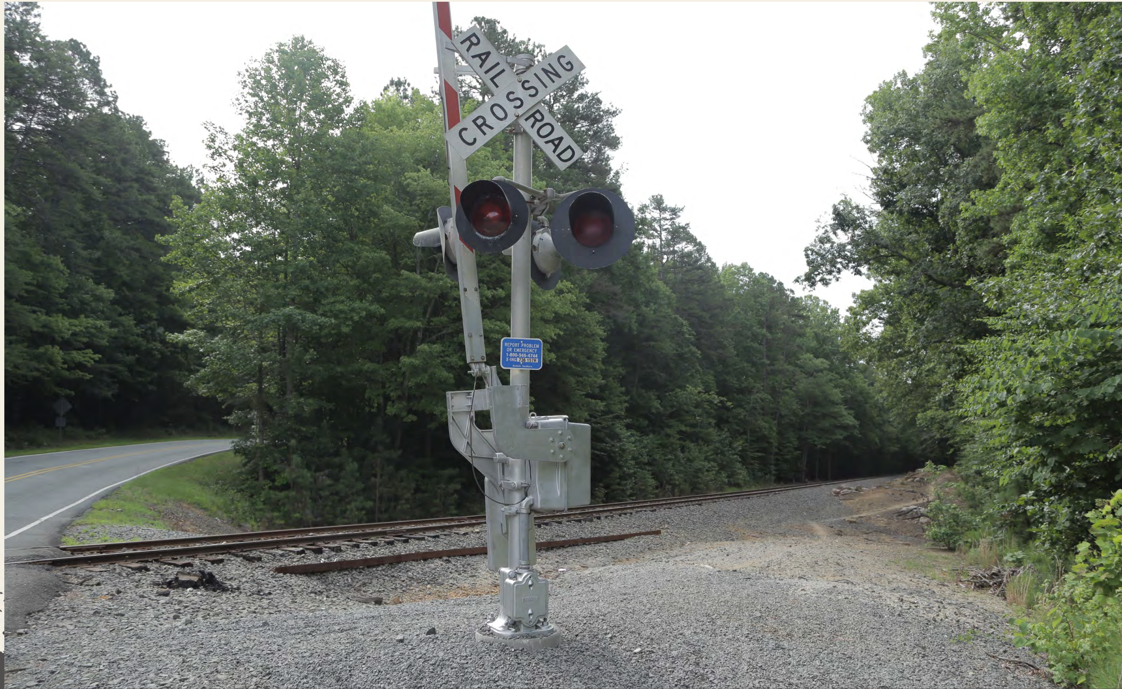
Railroad at Seawell School Rd Crossing
